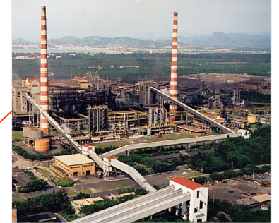
3BFs and 3 BOFs; 7.5Mt of annual slab capacity; HSM with 4.3Mt capacity
