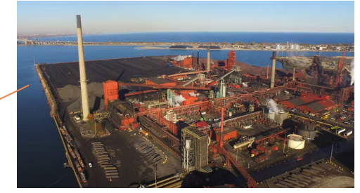
Dofasco, Canada, transitioning 2.5Mt of capacity to DRI and 2.4Mt to EAF by 2028
