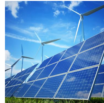
Renewable energy generation
