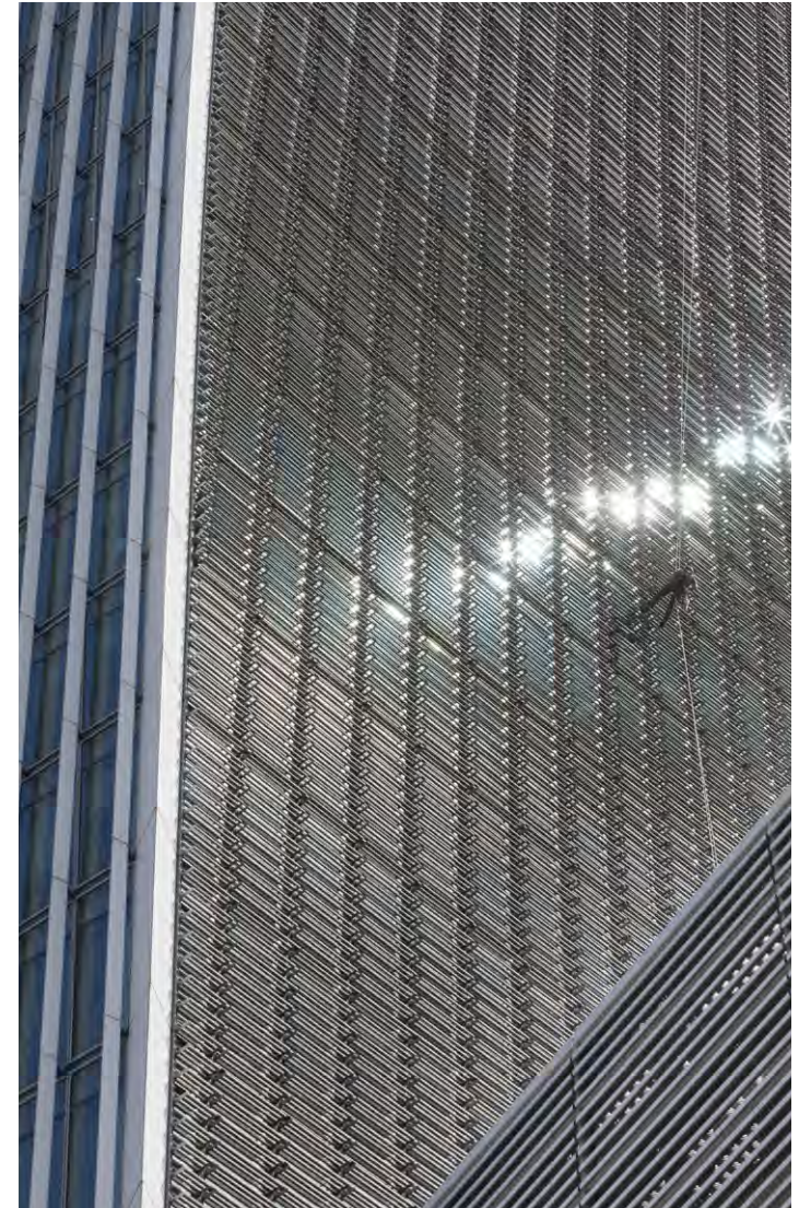
20 Fenchurch Street, London, United Kingdom
